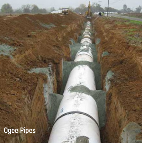
Spigot & Socket with Rigid Joint Pipes
